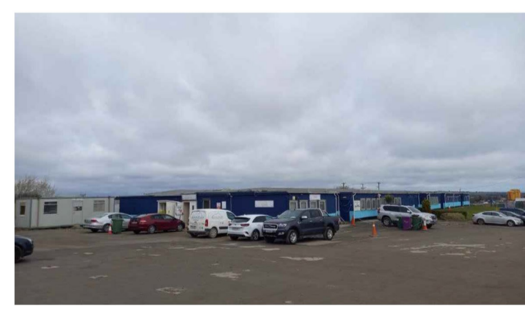
Photo: Current condition and use of the prefab buildings as temporary site office/site compound
